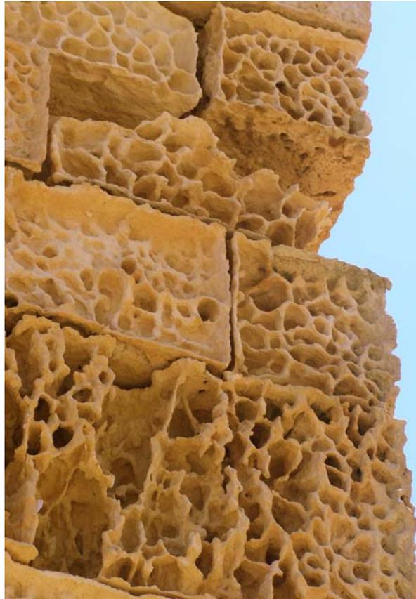
**Figure 1.** Honeycomb weathering of a limestone in Malta resulting from salt weathering that typically creates hollows, allowing salts to concentrate.
